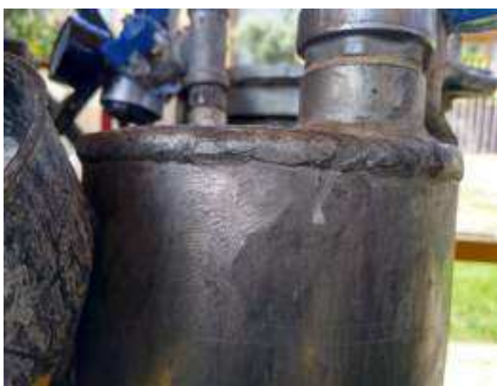
Solda do tampo superior
